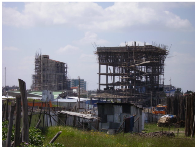
Picture 4: Construction site in Addis Ababa
